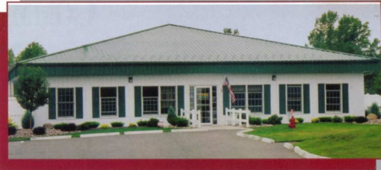
▲ Custom architectural design flexibility to blend into the local community.
